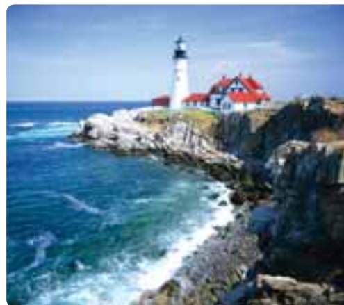
Portland Head Lighthouse, Maine
